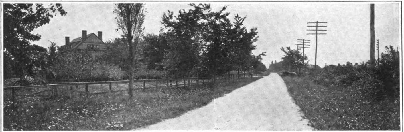
LOOKING SOUTH ON THE MASSAPEQUA ROAD CLOSE TO THE BETHPAGE TURNPIKE—AUTOMOBILE ON THE RIGHT IS MAKING THE TURN, WHICH IS MARKED BY THE HOUSE ON THE LEFT.
